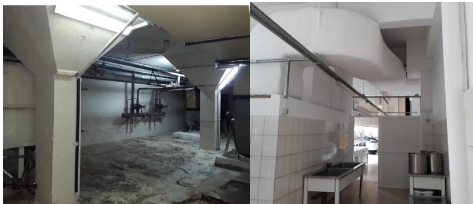
Figure 20 - Interior building system of the non-retrofitted canteen
